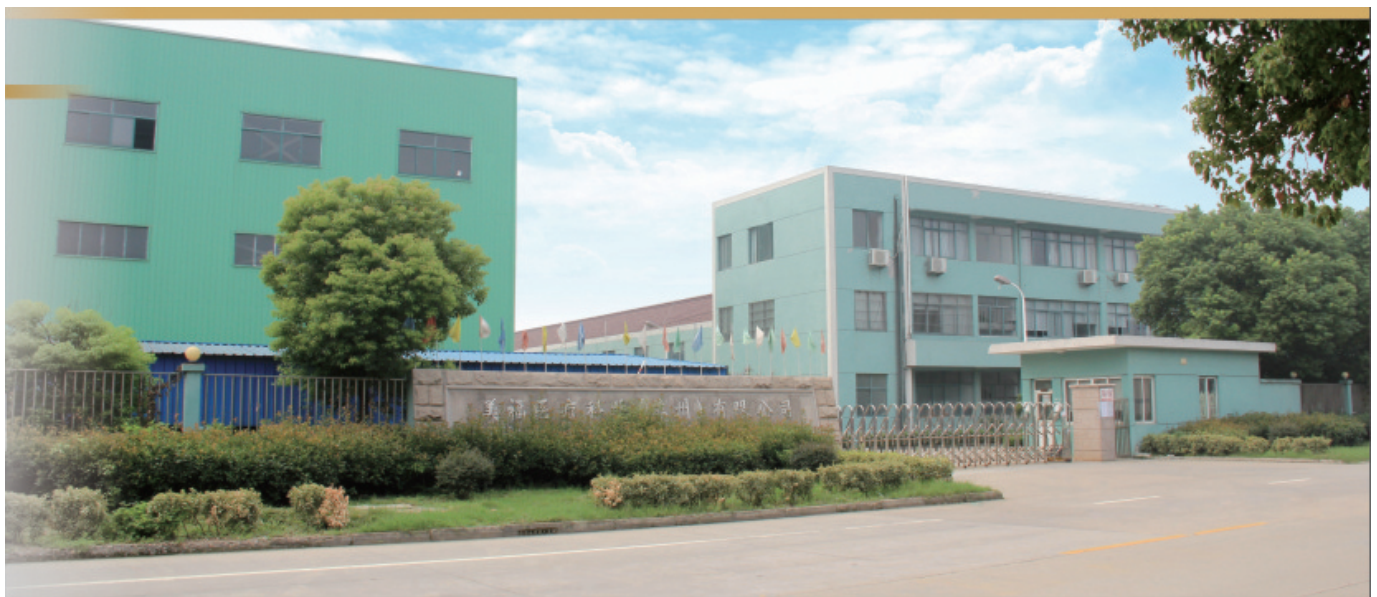
MeiFu Facility, Wujiang City, China
