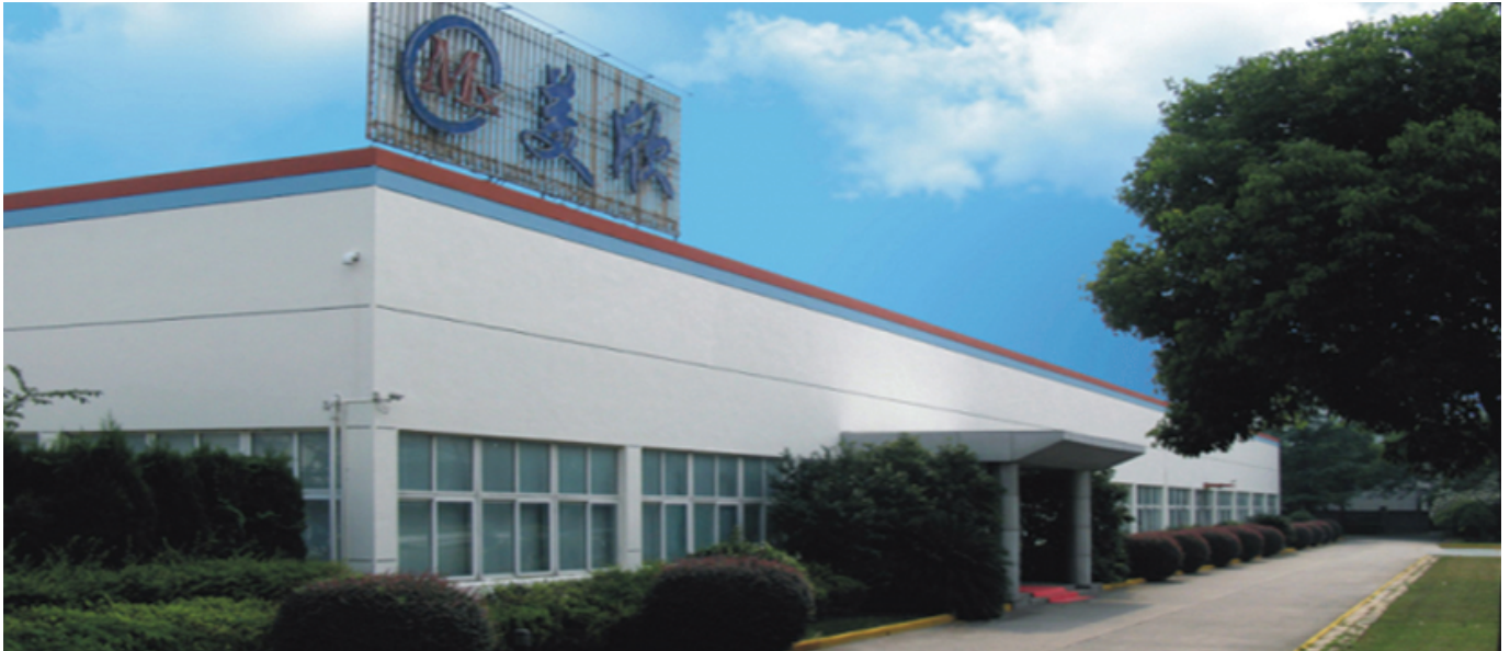
MeiXin Facility, Wujiang City, China
